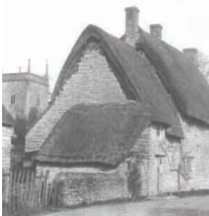
Original thatched roof of Mulberry Cottage.
