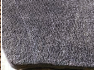
Thatch with protective mesh.
