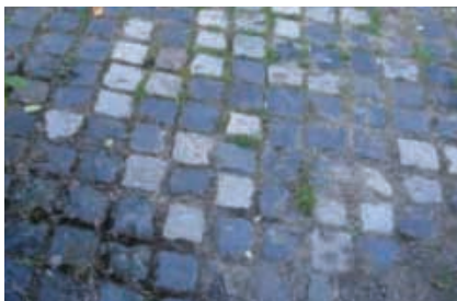
Granite setts used in private driveway
