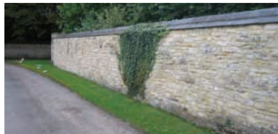
Boundary wall of the Vicarage with grey ridge tiles.
