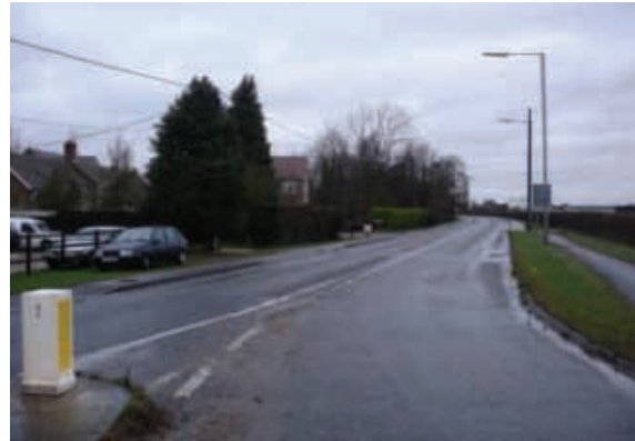
View north of B430 and junction with A34.
