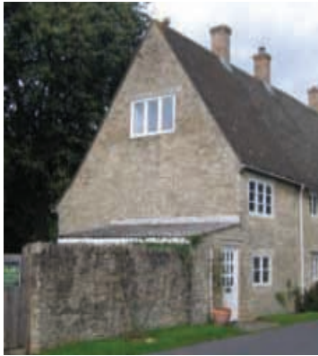
Existing steeply pitched roof of Mulberry Cottage.
