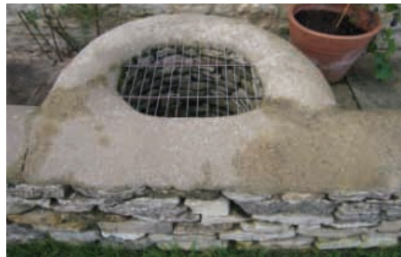
Well outside bungalow adjacent to Mulberry Cottage.
