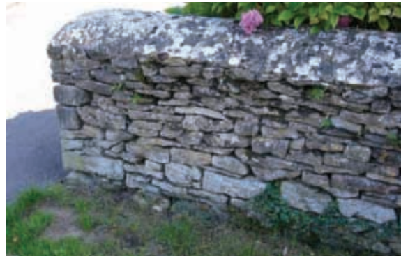
Heaped mortar forms coping
