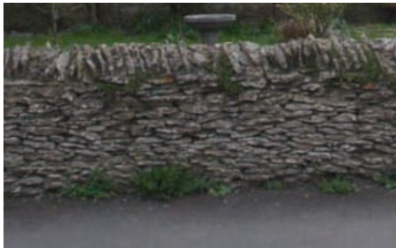
Boundary wall of Rutland Cottage.
