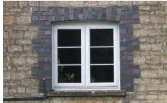
Vitrified brick detailing.
