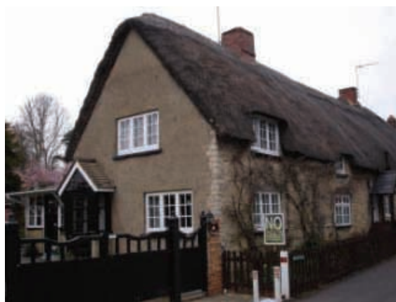
The Cottage, Church Lane with rendered flank wall.
