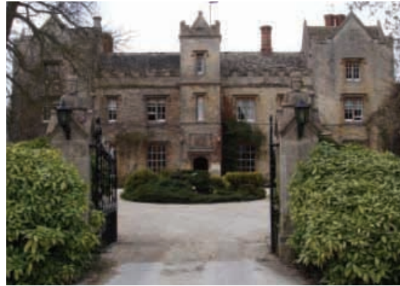
Pillars at the entrance to Weston Manor.
