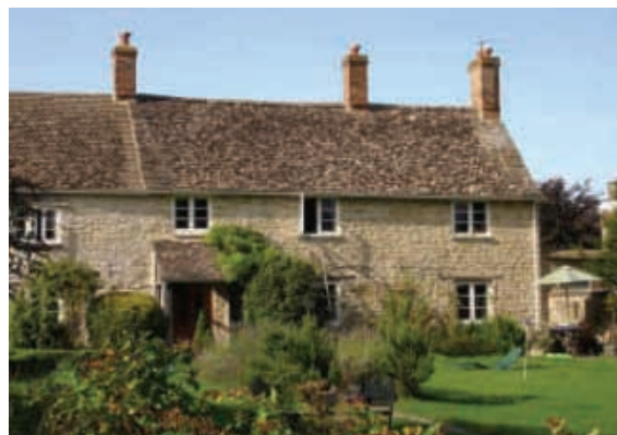
Southfield Farm Barn conversion.
