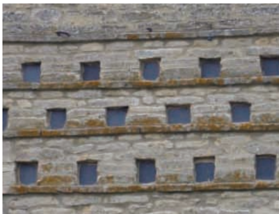
Stone gable wall of converted barn with in filled doves holes.
