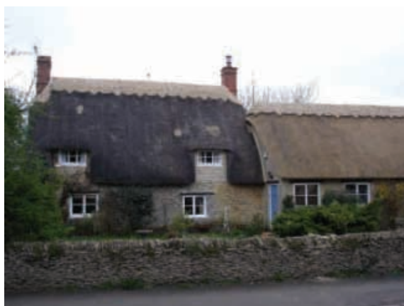
Rutland Cottage with newly thatched roof.
