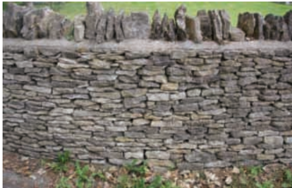
Stone laid on edge forms coping
